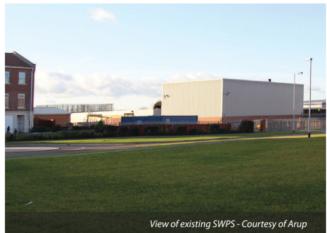
Existing SWPS building - Courtesy of Arup
